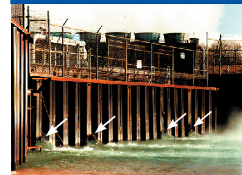
Water discharge area at a nuclear power plant on Lake Michigan. Note the flow from four big ejection outlets.
