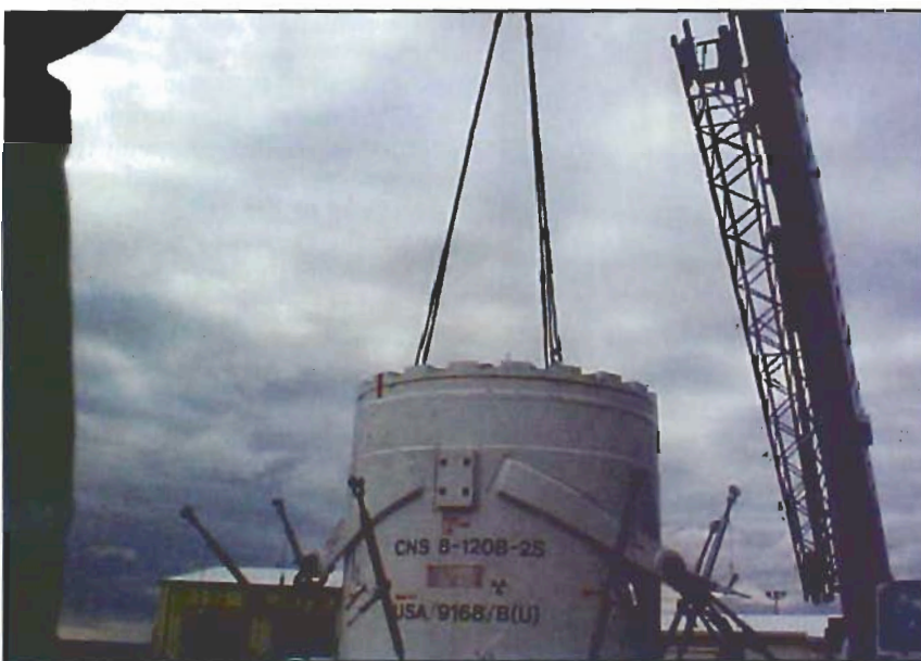
Unloading an LLW transportation cask at the WCS site.
