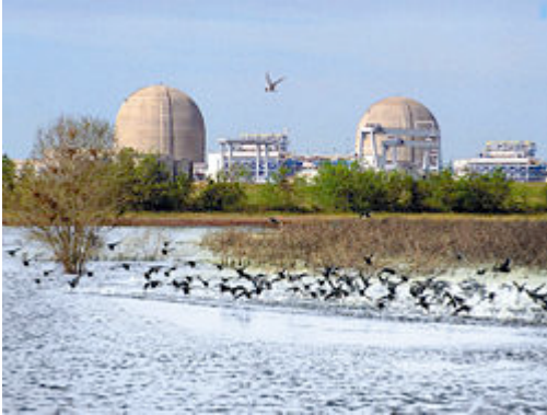
NRC Image of South Texas Project, Units 1 & 2.
